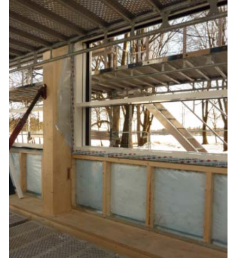
Good thermal insulation and air tightness. Photo: Skanska
