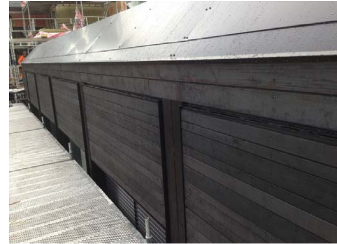
New cladding of burned wood/aspens (giving black surface), Photo: Skanska
