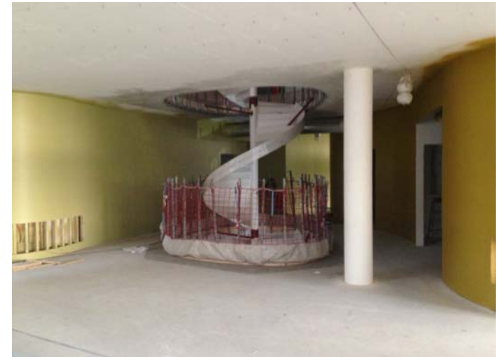
Exhaust air via open stairwells. Photo: Skanska
