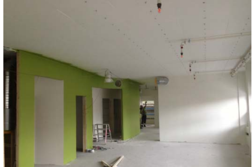
Exposed thermal mass in ceiling. Photo: Skanska
