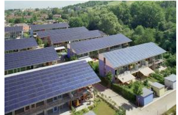
Solar Settlement Freiburg, Germany Architecture and Concept: Rolf Disch
