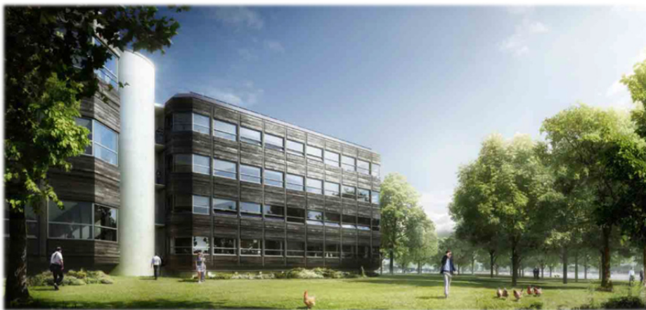
Figure 43 Powerhouse Kjørbo, Sandvika (Energirapporten 9/36, 2013).
