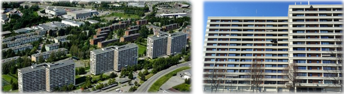
Figure 32 Tveitta Borettslag, Oslo, Norway.
