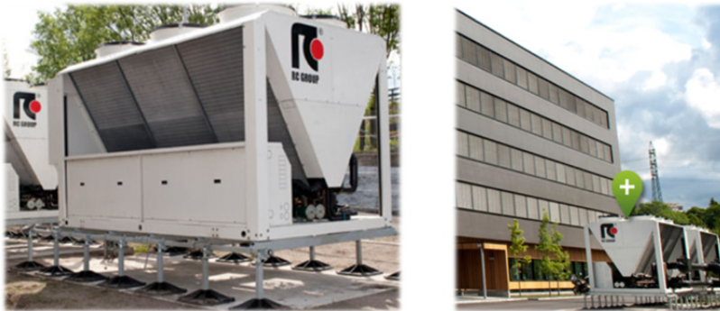
Figure 31 The reversible air-to-water heat pump and chiller units (GK Norway, 2013).
