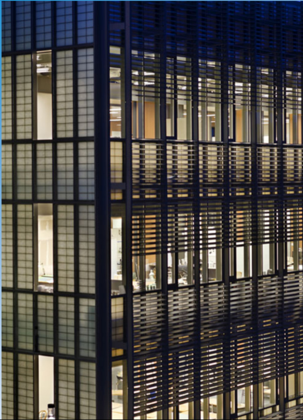
Translucent aerogel in use in Sculpture Building and Gallery of Yale University, New Haven, Connecticut, USA.
