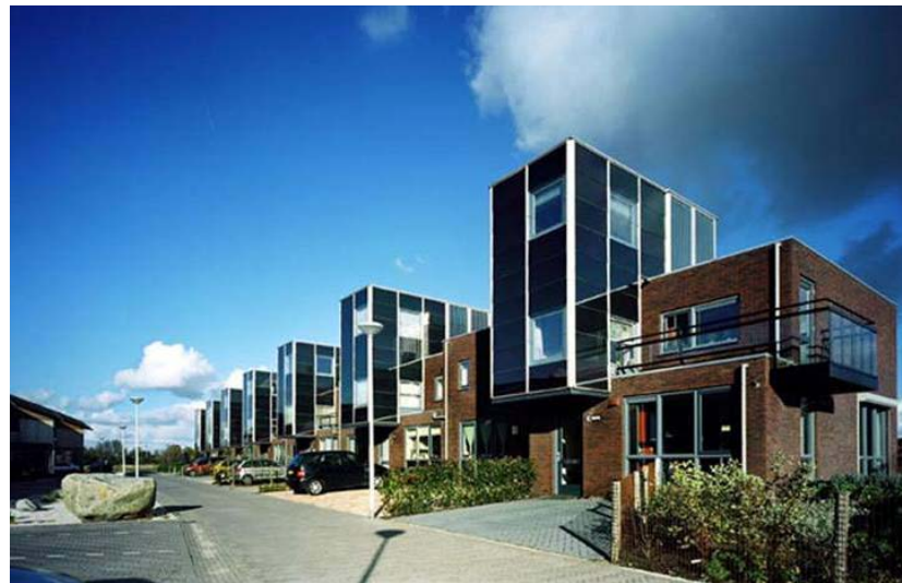
PV panels on the facade of row houses, Netherlands. Source: Kiss&Cathcart Gregory Kiss
