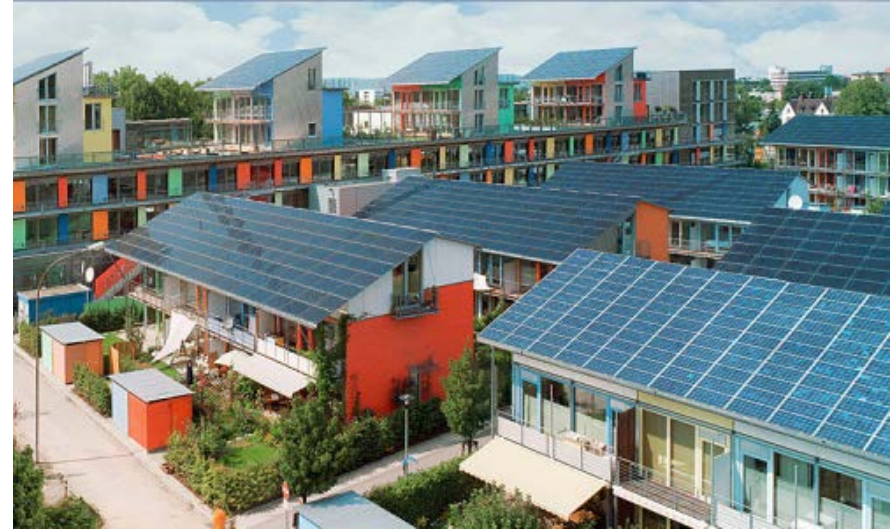
Plus energy settlement in Freiburg. Source: iea40.buildinggreen.com
