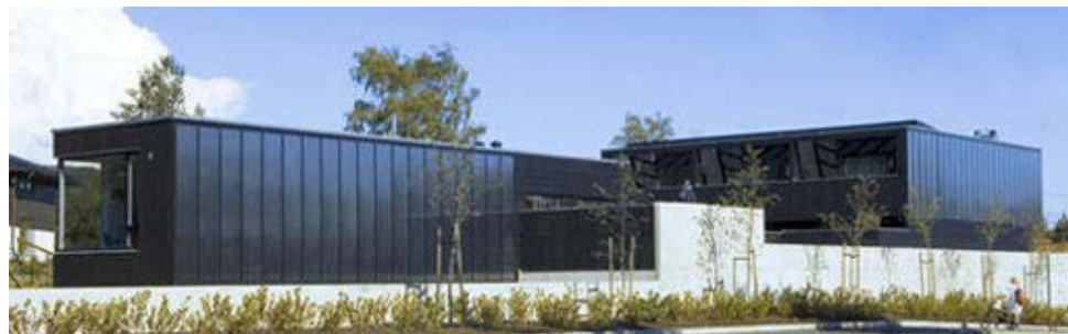
Housing project with solar thermal collectors in the facades, Oslo. Source: SOLARNOR
