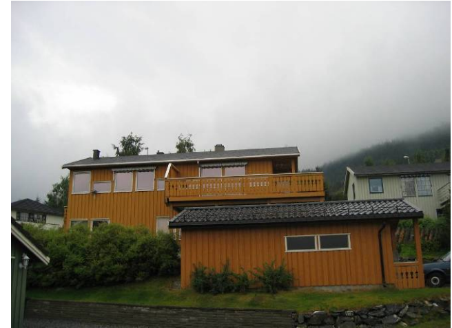
Single house in Orkanger, renovated to low-energy standard
